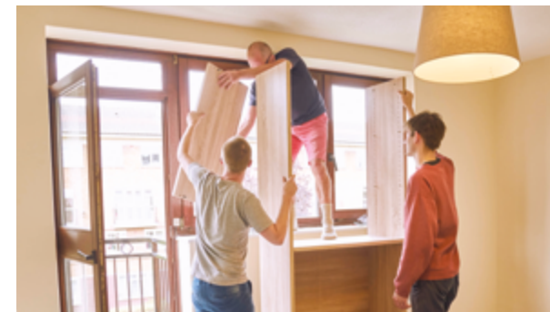
Preparing one of the flats in the project
